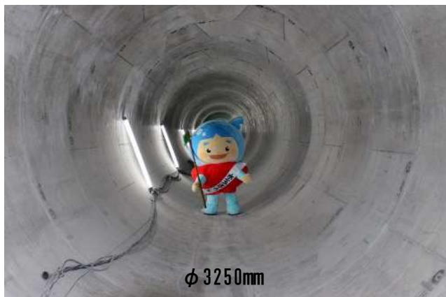
【大石2号貯留管】貯留量16,700m 3
